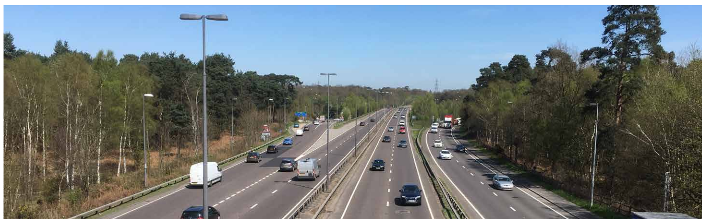
View northeast from Cockcrow bridge towards junction 10, showing the woodland surroundings to the A3
