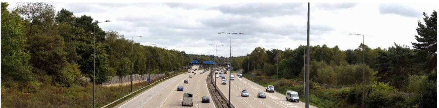
View west from Clearmount bridge towards junction 10, with noise barriers along the wooded edges of Wisley Common
